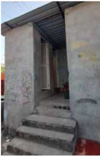
Toilet Facility for workers
